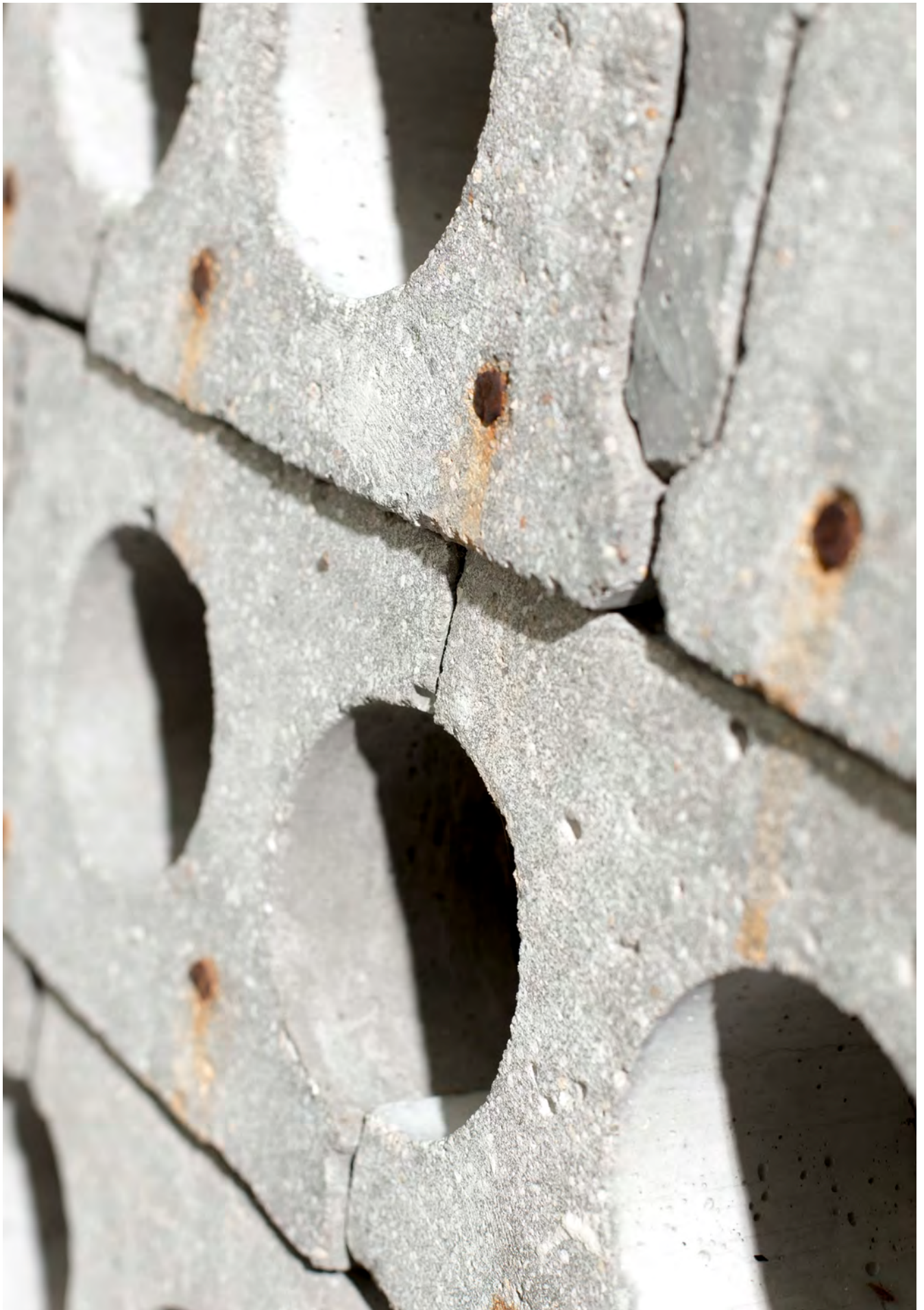
Figure 23/ Detail of facade prototype from sliced concrete slabs. The weathering from reinforcement bars adds character to the surface
