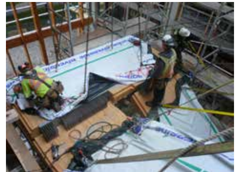
The 'free-floating' staircase connection to the landing using the Holz-Stahl-Komposit-Systeme (HSK-System)™. This system uses glue to connect the steel members to the wood. Photo Credit: Equilibrium Consulting Inc.
