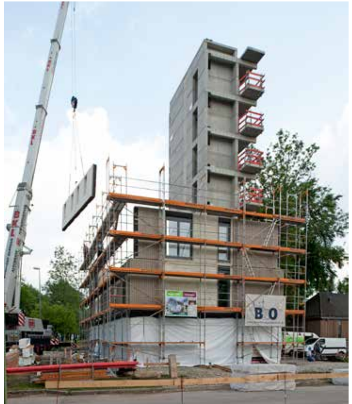
Left: Prefabrication of wall panels. Right: Timber erection time took 2 days per level. Photo credit: Huber&Sohn
