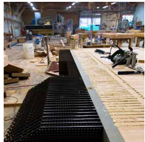
Installation of HSK perforated steel connectors. Photo Credit: Equilibrium Consulting Inc.
