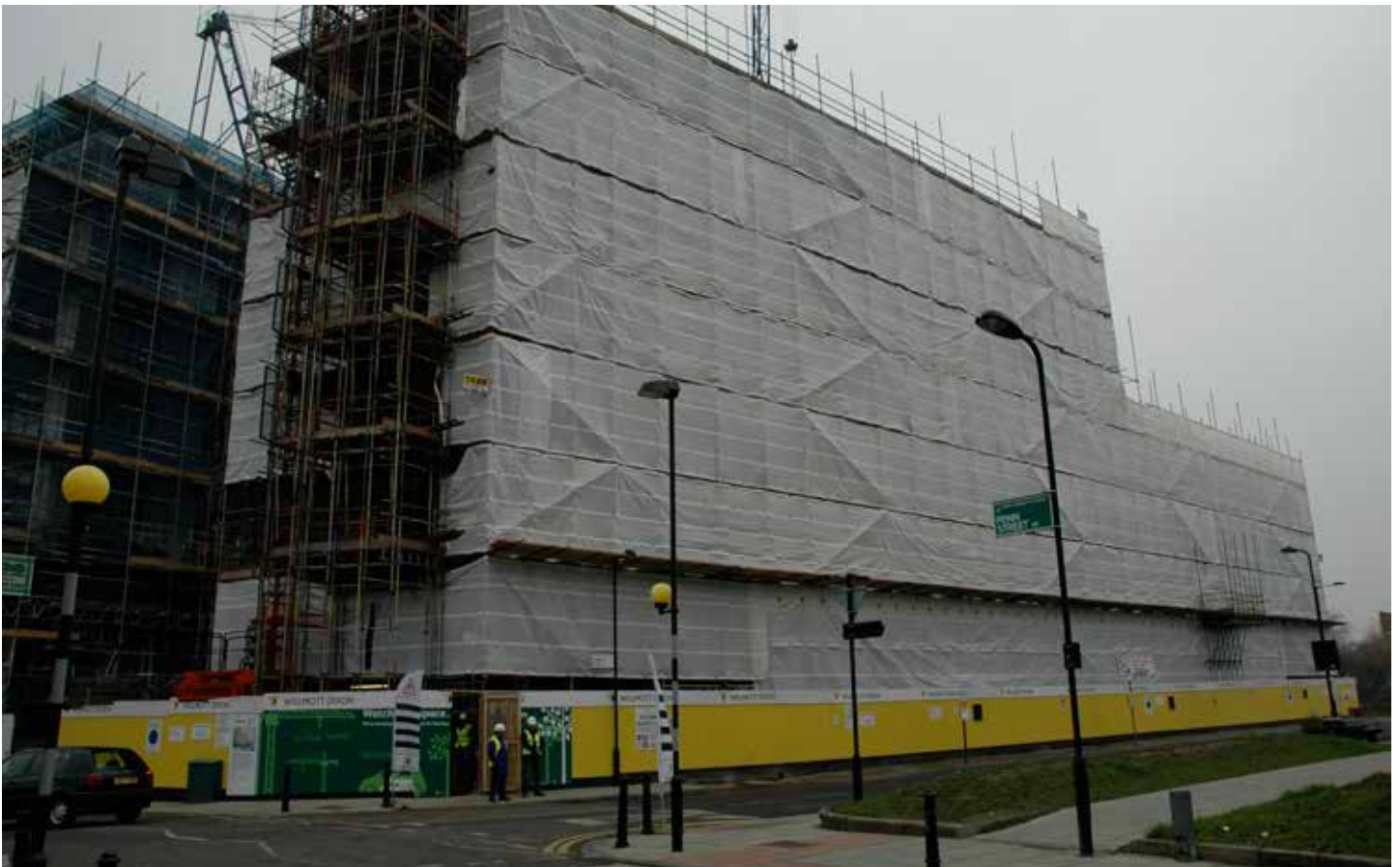
Façade enclosed during construction. Photo credit: Willmott Dixon Group
