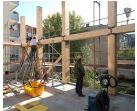
Timber structural frame Photo Credit: Architecture by Kaden Klingbeil, Photo by Bernd Borchardt
