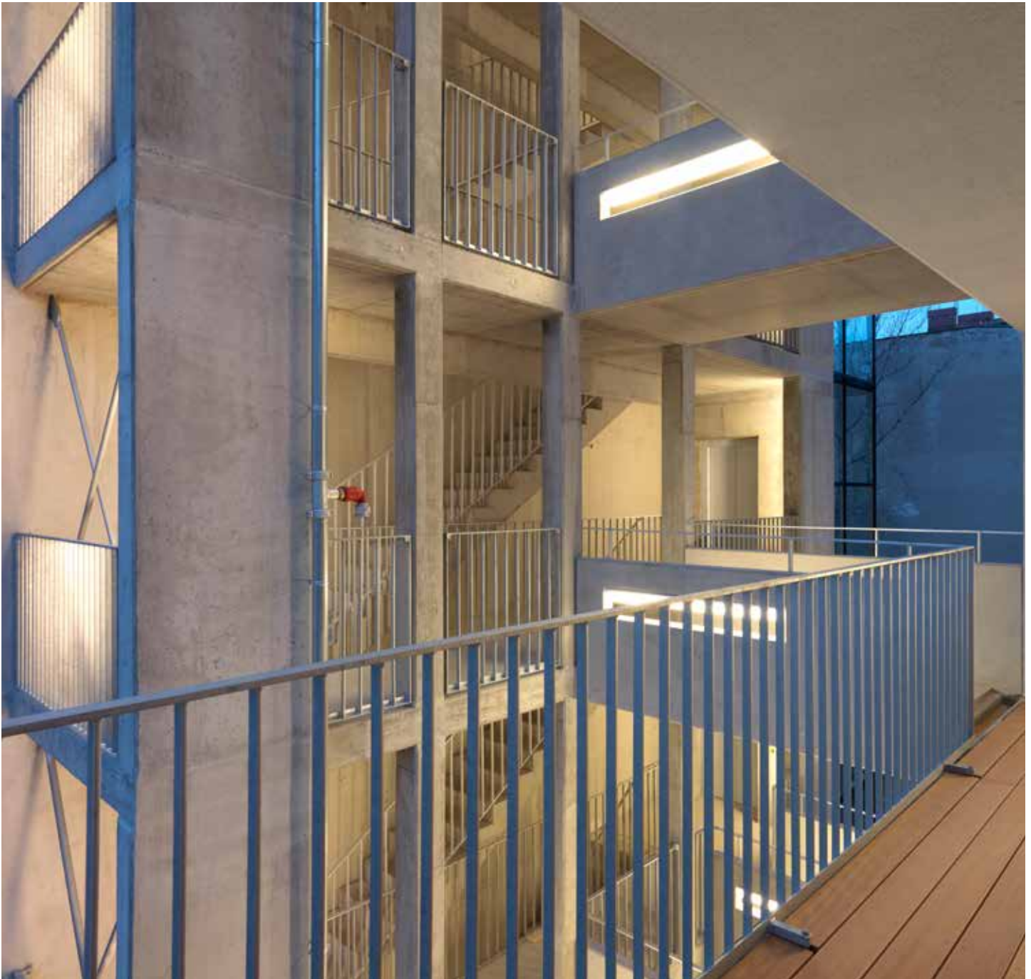
Exterior concrete stair and elevator shaft. Photo Credit: Architecture by Kaden Klingbeil, Photo by Bernd Borchardt
