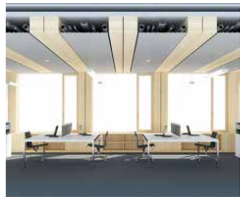
Systems are concealed behind aluminum panels within ceiling cavities. www.creebuildings.com
