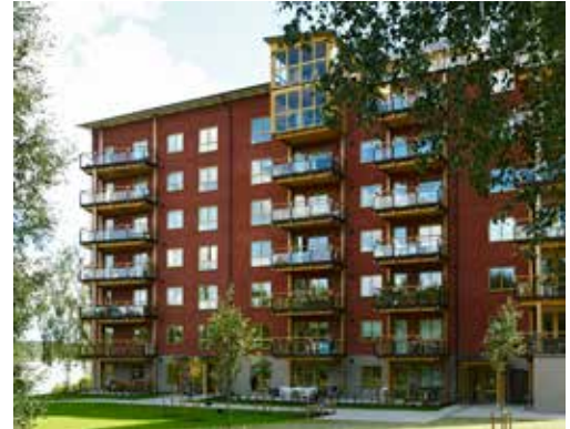
Non-combustable exterior cladding, north façade. Photo Credit: Midroc Property Development
