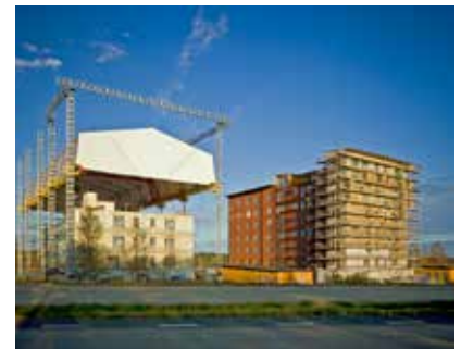
Movable, rising tent for weather protection during construction.
