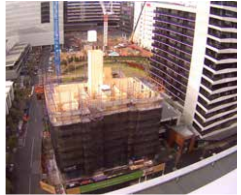
Dust protection sheet surrounding the scaffolding. Photo credit: Lend Lease
