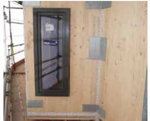
CLT floor panels and walls secured with custom gang nail steel plates. Photo credit: Willmott Dixon Group
