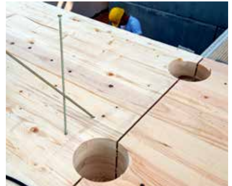
Cross screw technique used to connect floor and wall panels. Photo credit: Huber&Sohn
