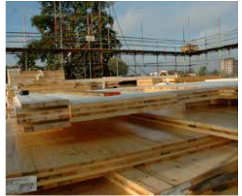
Cross laminated timber panels stored on-site Photo credit: Willmott Dixon Group
