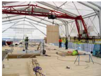
Weather protection at Limnologen. Moveable rising tent structure. Photo credit: Johan Vessby
