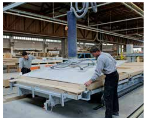
Prefabrication process. Photo credit: Huber&Sohn
