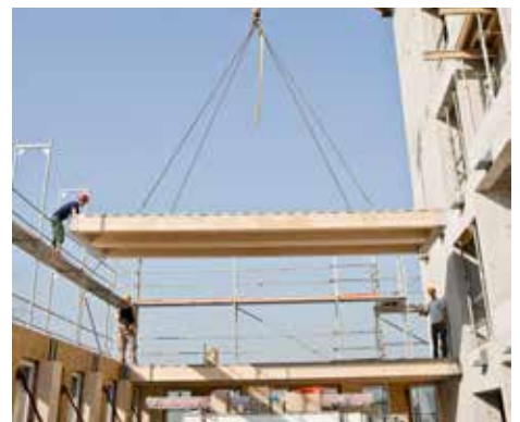
Installation of hybrid floor slab. Photo Credit: www.creebuildings.com
