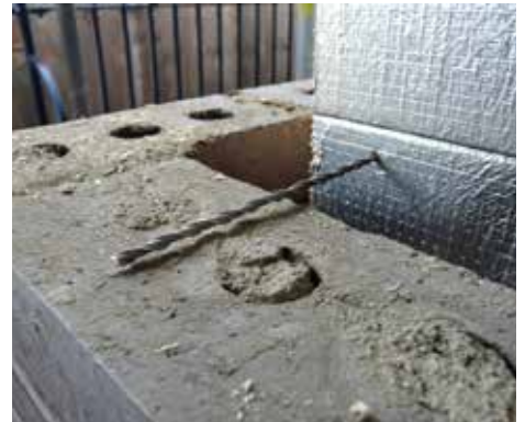
The solid external wall panels are ideally suited to helical brick ties. Photo credit: Willmott Dixon Group
