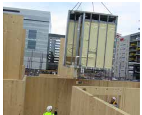
Installation of prefabricated bathroom pod Photo credit: Lend Lease
