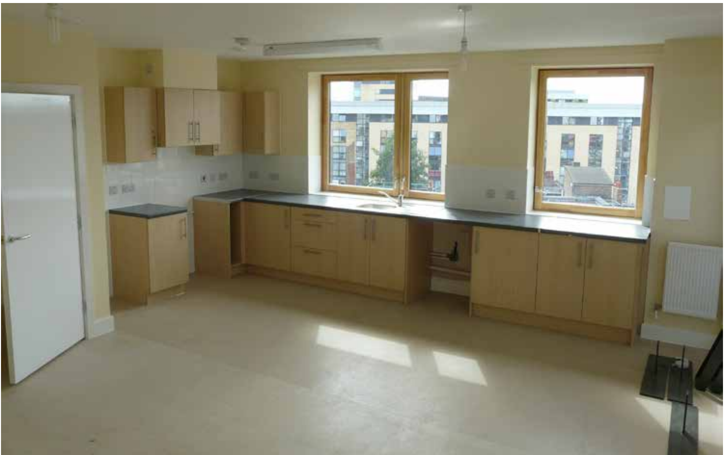
Interior of residential suite. Photo credit: Willmott Dixon Group
