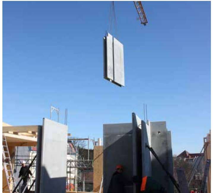
Installation of precast concrete panels Photo credit: Rozynski Sturm Architekten
