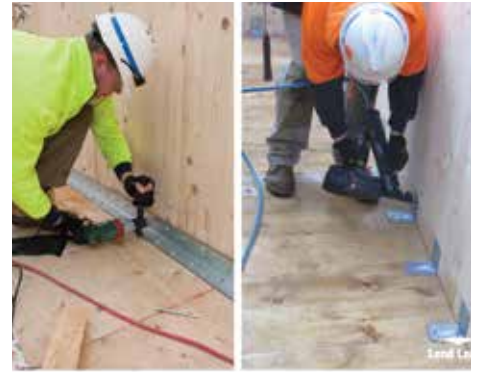
Angled steel connection plates and screws. Photo credit: Lend Lease
