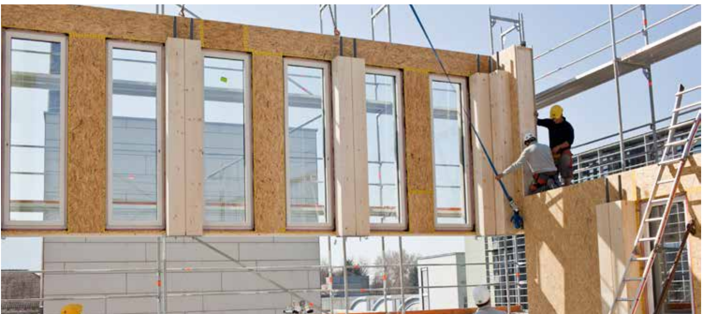
Installation of prefabricated wall panels. Photo Credit: www.creebuildings.com
