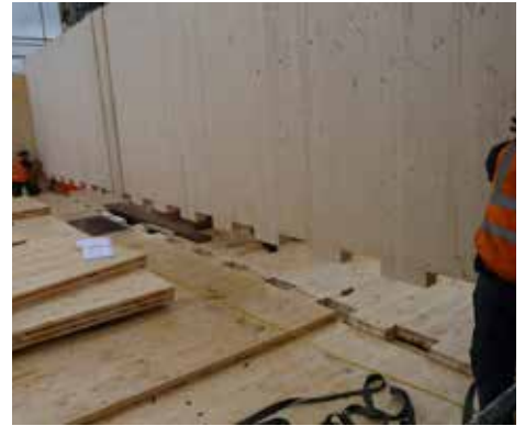
Interlocking keyed edge of each floor and wall panel. Photo credit: Willmott Dixon Group
