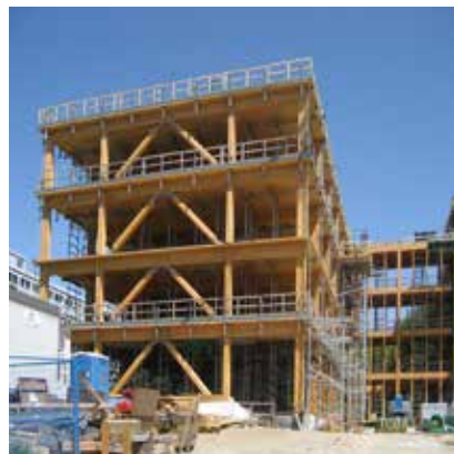
Exposed view of glulam chevron braces at UBC Earth Sciences Building Architecture by: Perkins+Will Photo credit: Equilibrium
