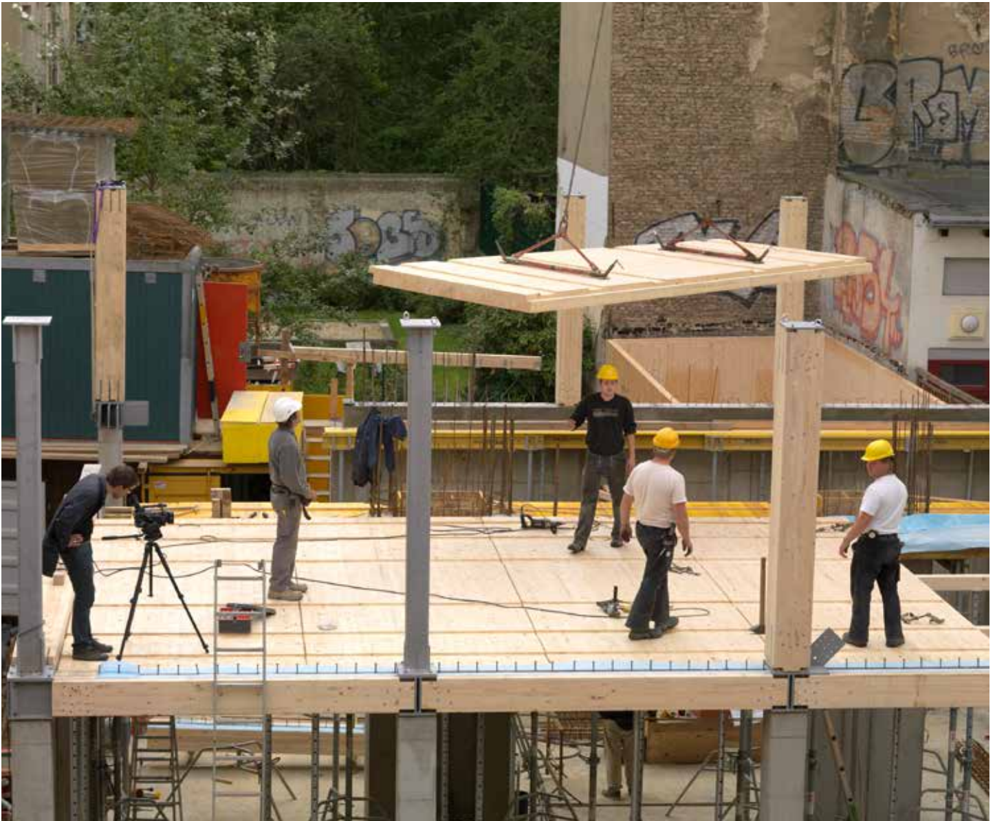
Installation of CLT floor panels Photo Credit: Architecture by Kaden Klingbeil, Photo by Bernd Borchardt
