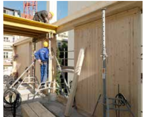
Brettstapel exterior walls in place. Photo Credit: Architecture by Kaden Klingbeil, Photo by Bernd Borchardt
