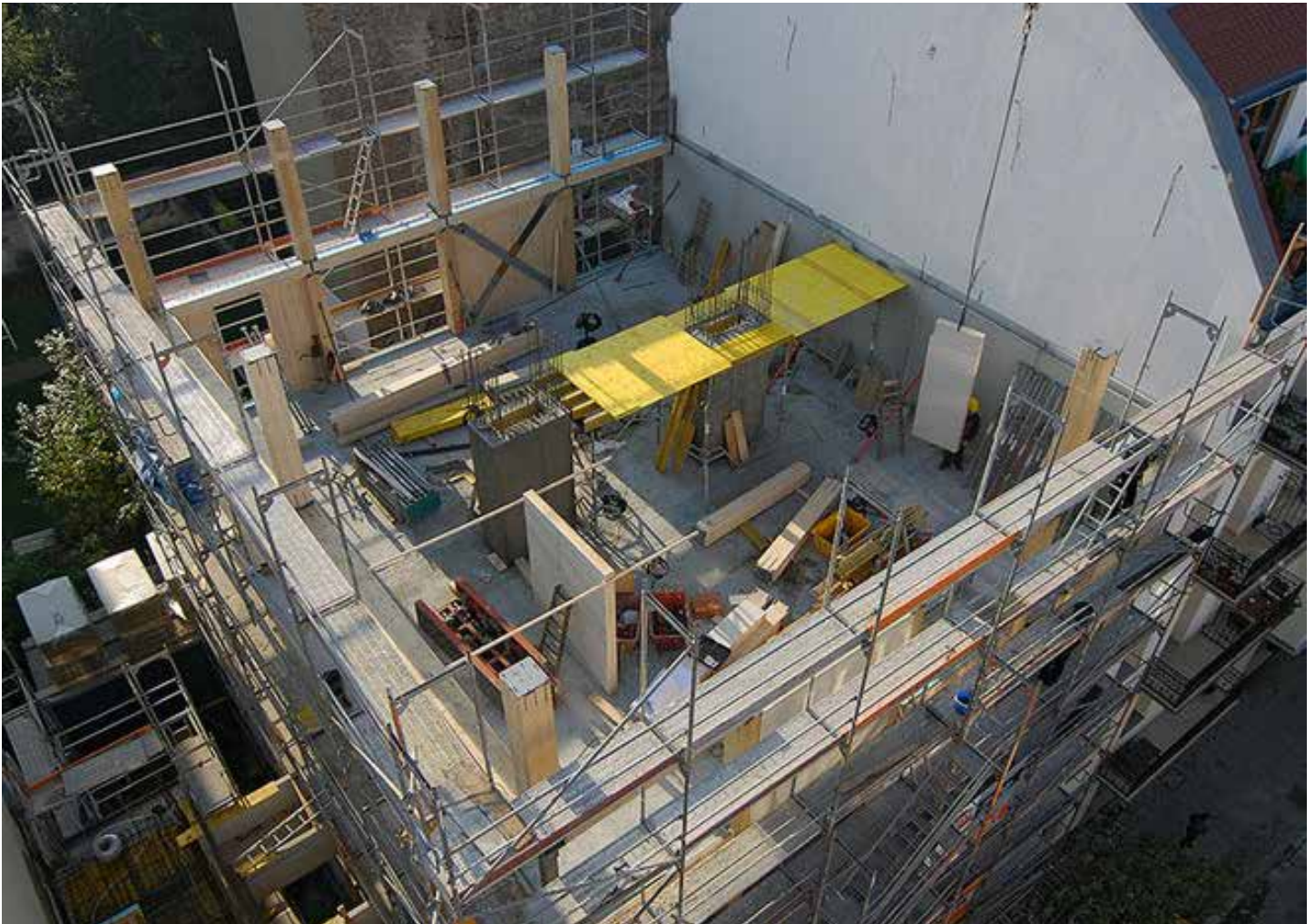
Aerial image during construction Photo Credit: Architecture by Kaden Klingbeil, Photo by Bernd Borchardt
