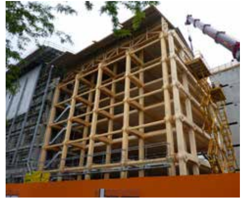
Temporary roof over timber structure Photo Credit: Shigeru Architects
