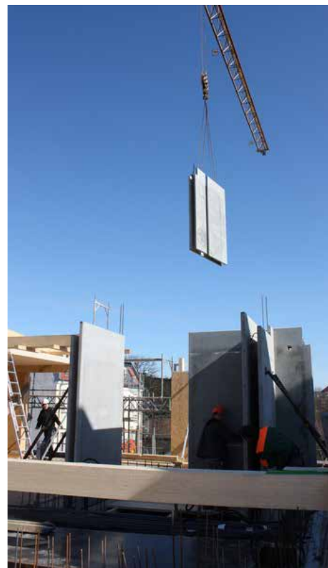
Installation of precast concrete element at 3XGRÜN Photo credit: Rozynski Sturm Architekten
