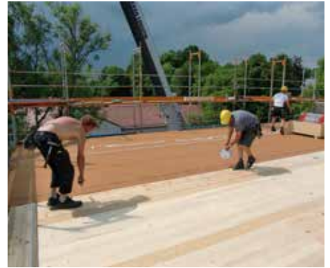
Floor panels covered with waterproof membrane after installation. Photo credit: Huber&Sohn
