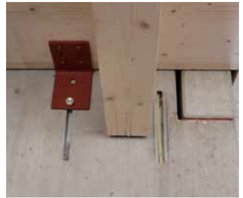
Steel bracket used to connect wood floor panels to concrete core. Photo credit: Huber&Sohn
