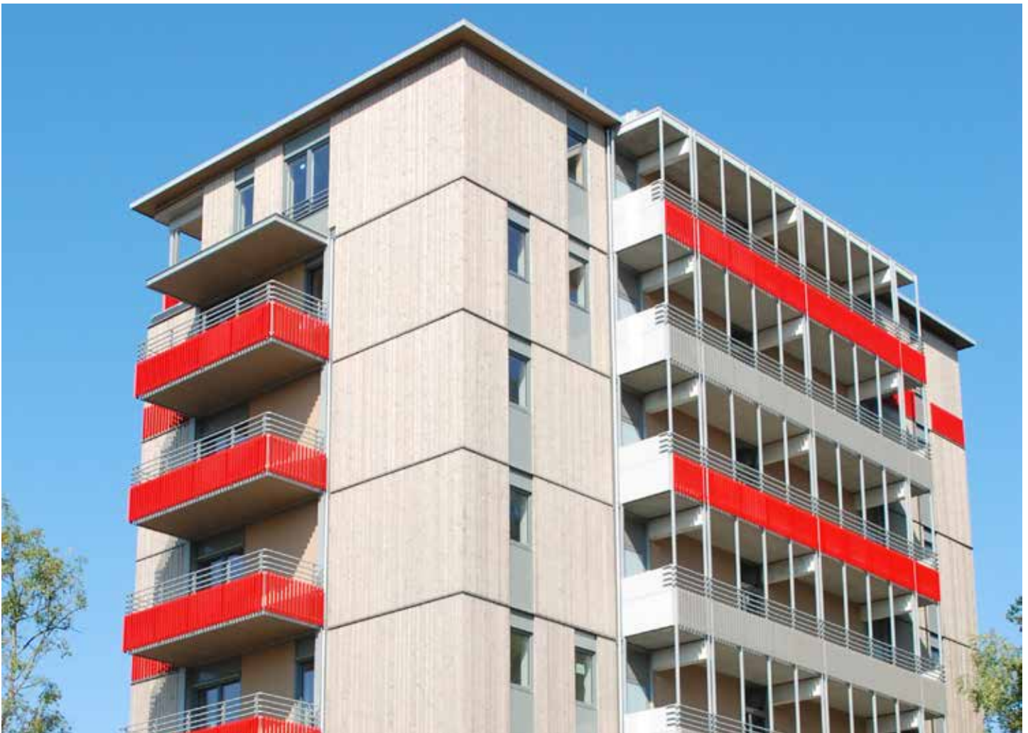
External concrete corridors provide smoke free escape route pictures. Photo credit: SCHANKULA Architekten / Photographer: Arthur Schankula
