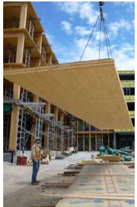
Lifting of CLT panel. Photo Credit: Equilibrium Consulting Inc.
