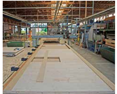
Prefabrication process. Photo credit: Huber&Sohn
