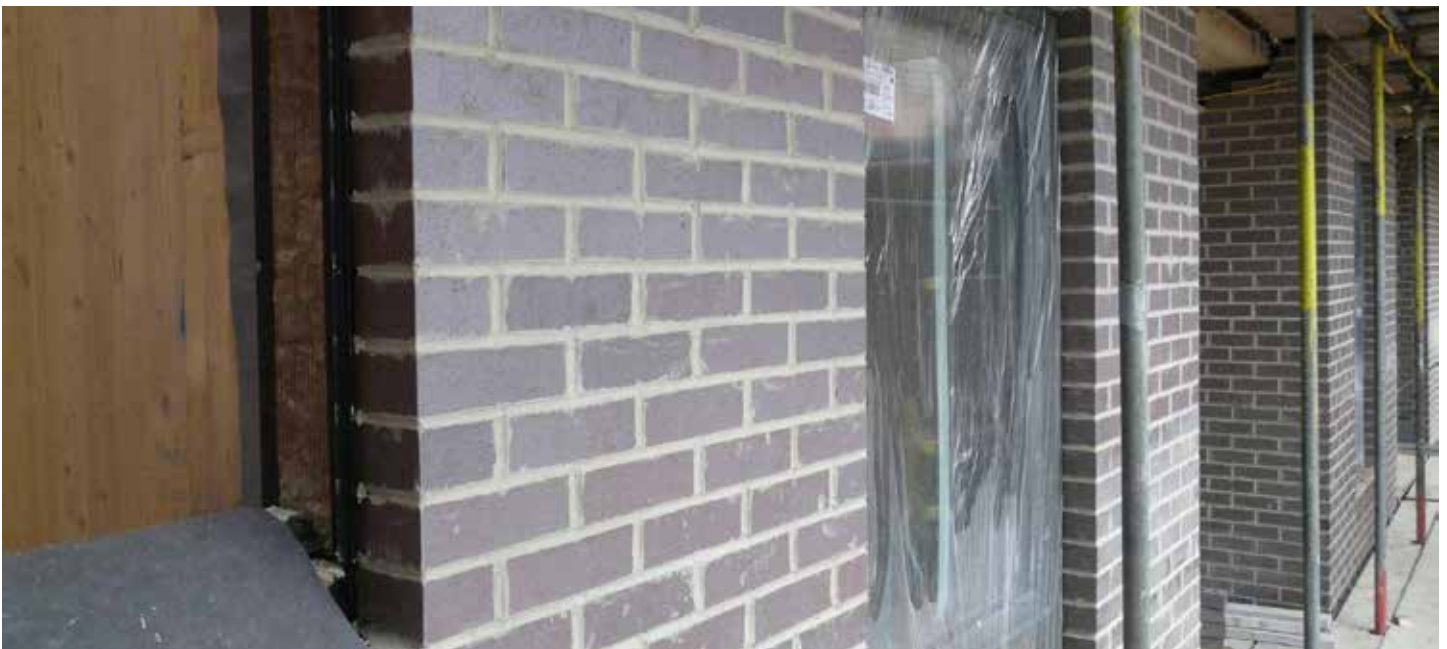
Exterior brick cladding. Photo credit: Willmott Dixon Group
