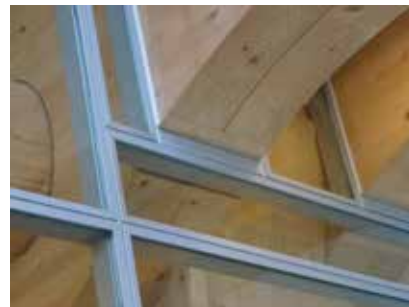
Notched interface conceals non-combustible barriers on timber beams at Tamedia. Architecture by: Shigeru Ban Photo credit: R. Holt
