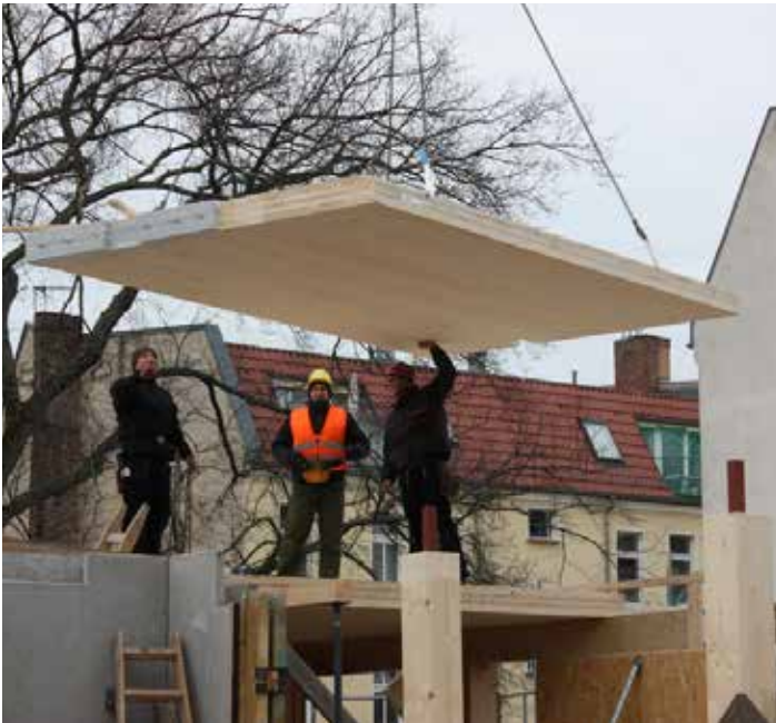
Installation of CLT floor panels Photo credit: : Rozynski Sturm Architekten
