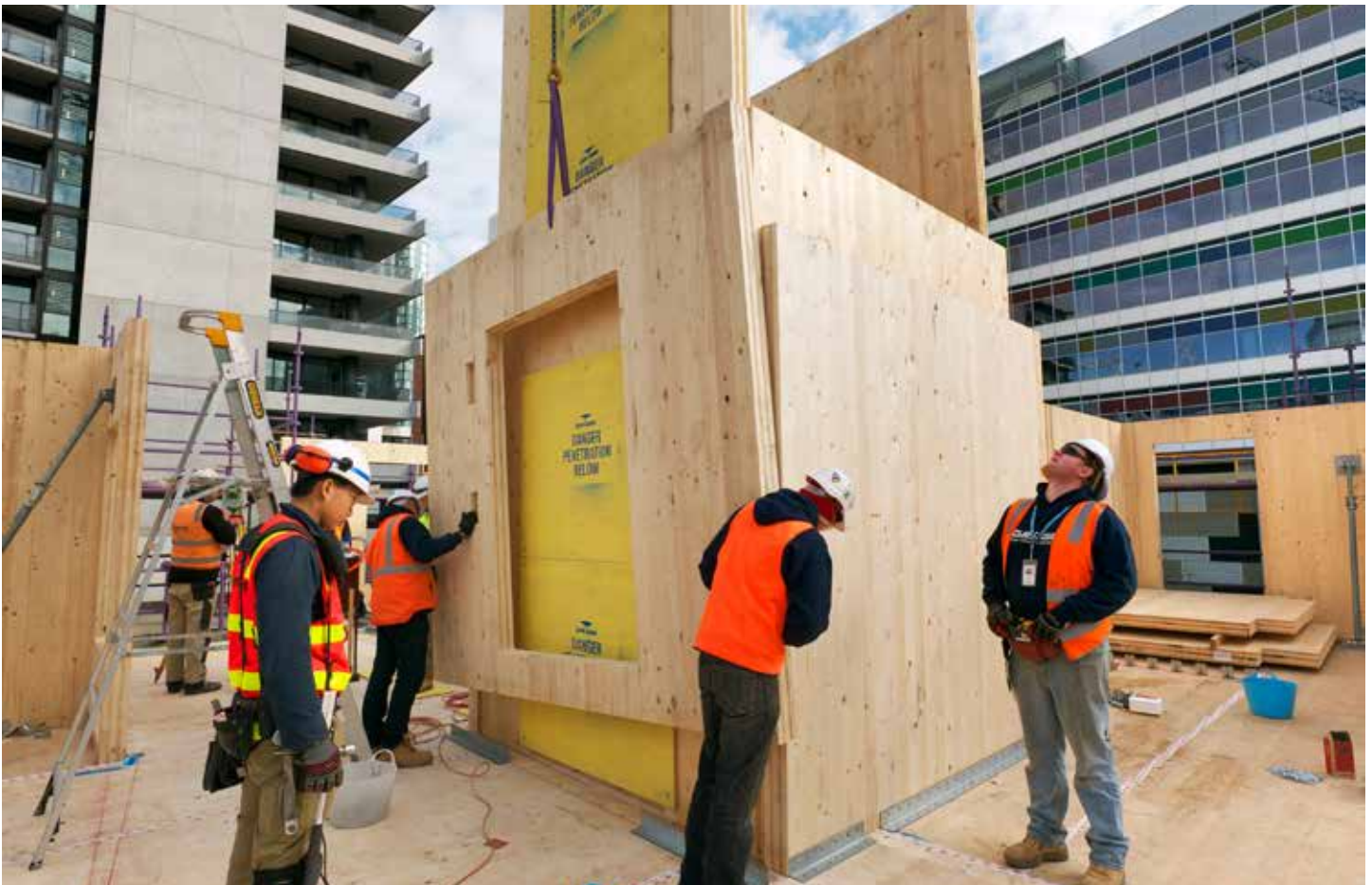
Installation of CLT elevator core Photo credit: Lend Lease
