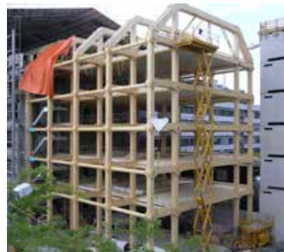
Tamedia post and beam structure Architecture by: Shigeru Ban Photo credit: Blumer-Lehmann AG
