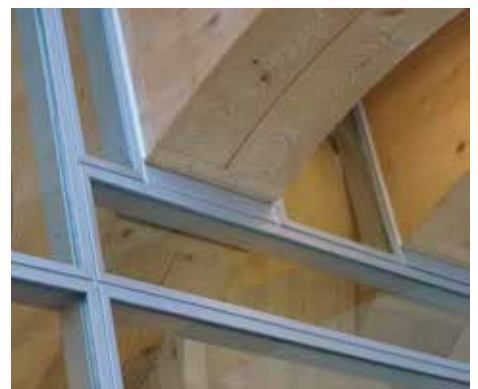
Notched interface conceals non-combustible barrier on timber beams Detail Credit: Rebecca Holt
