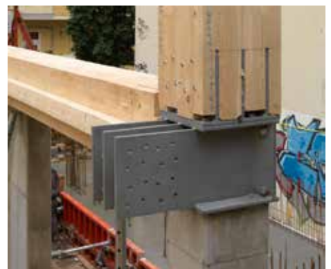
Steel connections. Photo Credit: Architecture by Kaden Klingbeil, Photo by Bernd Borchardt
