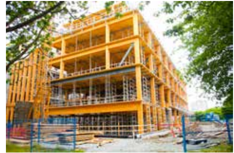
Significant scaffolding required on site. Photo Credit: K. K. Law
