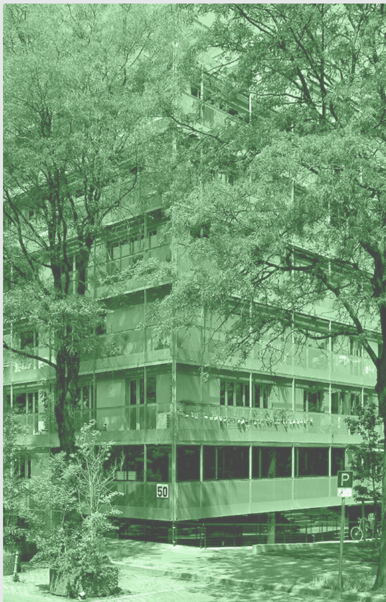
Photo of R50 Baugruppen
