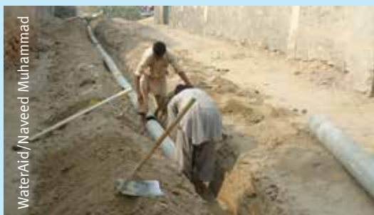
Installing sewer lines to connect sewage treatment units with household latrines in Muzafagarh, Pakistan
