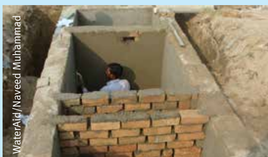
Sewage treatment unit under construction, Pakistan
