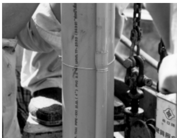
Figure 7.17 Use of small diameter pipe as centralisers
