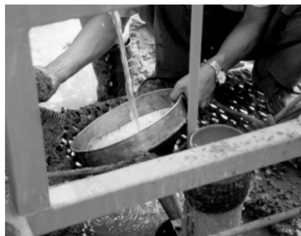
Figure 7.19 Gravel packing – note water flow up has stopped – gravel landed above screen level
