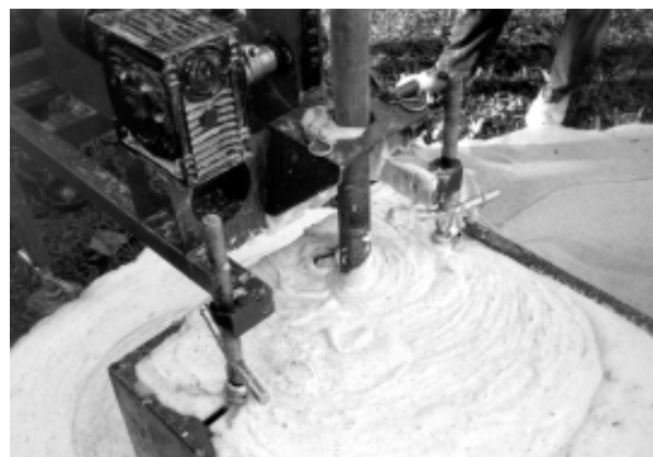
Figure 4.1 Drilling with stable foam
