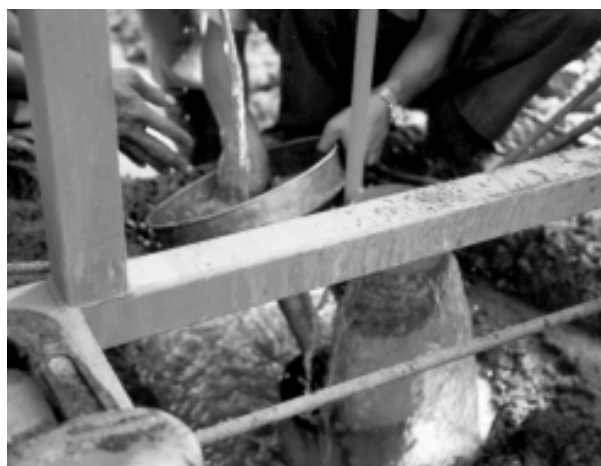
Figure 7.18 Gravel packing being added by funnel note water overflowing casing – gravel dropping below screened layer
