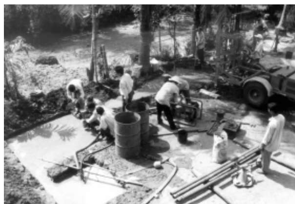
Figure 2.6 Functioning mud pits – slow moving flow for good settlement
