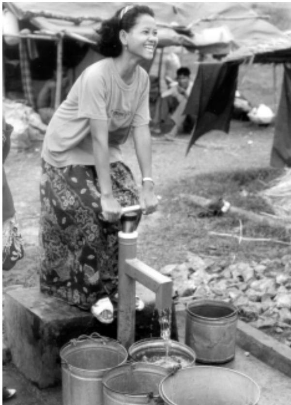
Figure 6.2 Direct Acting hand pump
