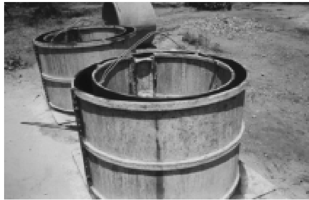
Photograph 11-2 - Formwork assembled and ready for use
