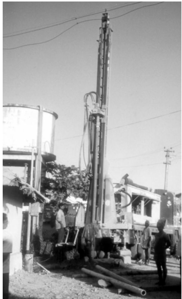
Photograph 4-2 - A rotary drilling rig
