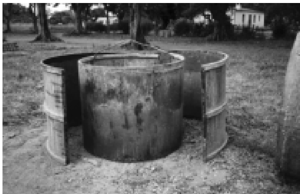
Photograph 11-1 - Inner and outer formwork, dismantled
