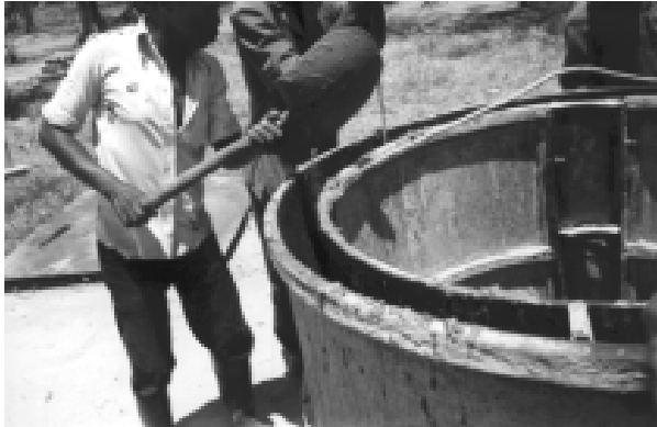
Photograph 11-3 - Pouring a ring
