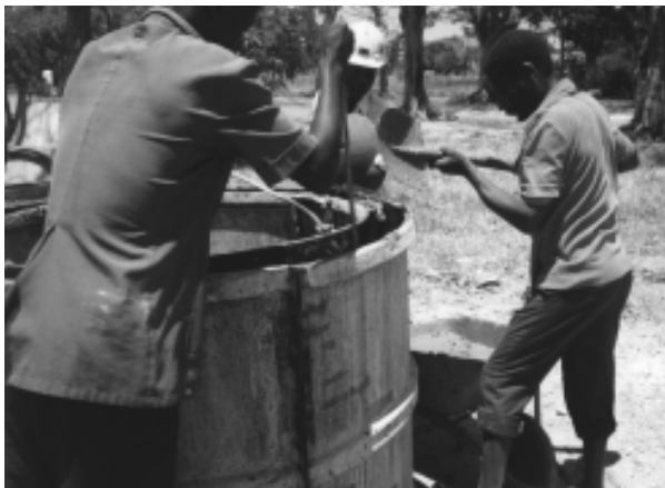
Photograph 11-4 - Rodding to ensure compaction
