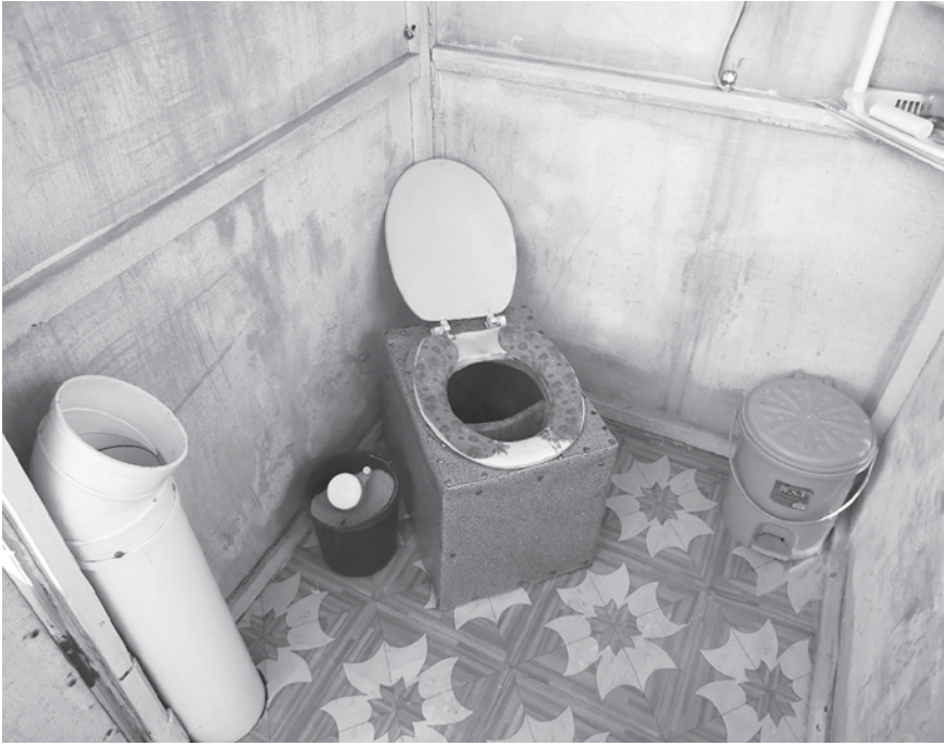
Figure 11.4 Toilet cubicle in a cold region
