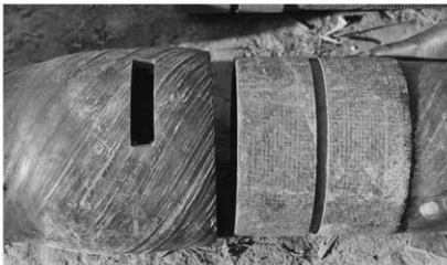
Glass Reinforced plastic joint
