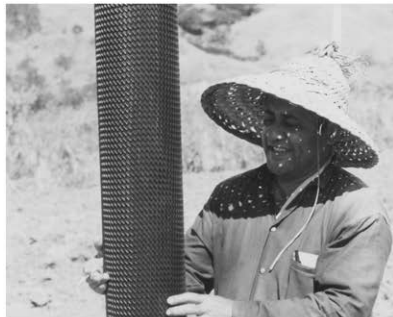
Geotextile wrapped slotted uPVC screen
