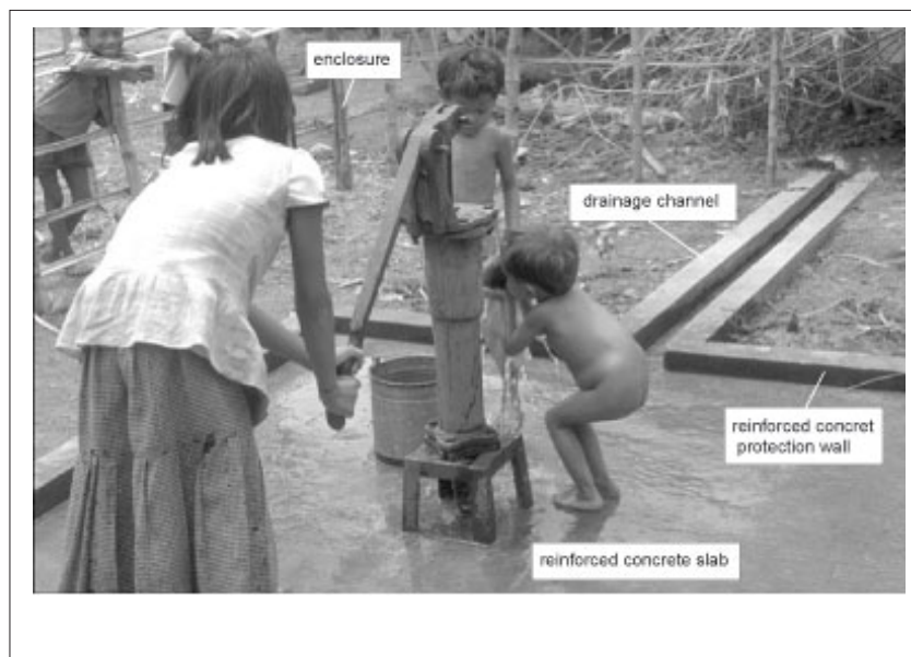
Figure 24: Important features of surface works for a borehole.
