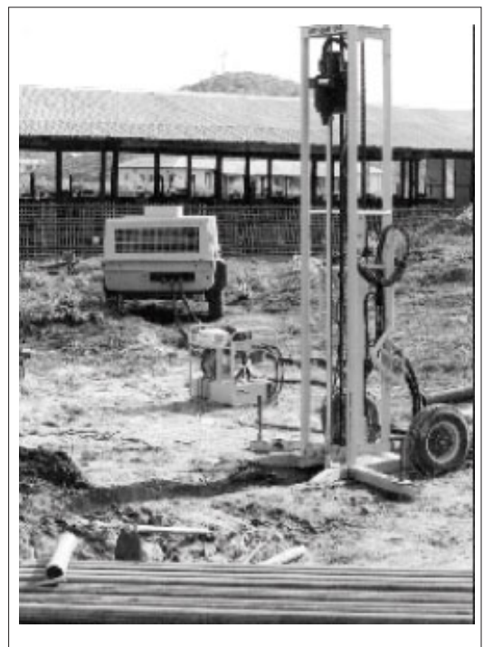
Figure 7: Rig, hydraulic pump, compressor.
