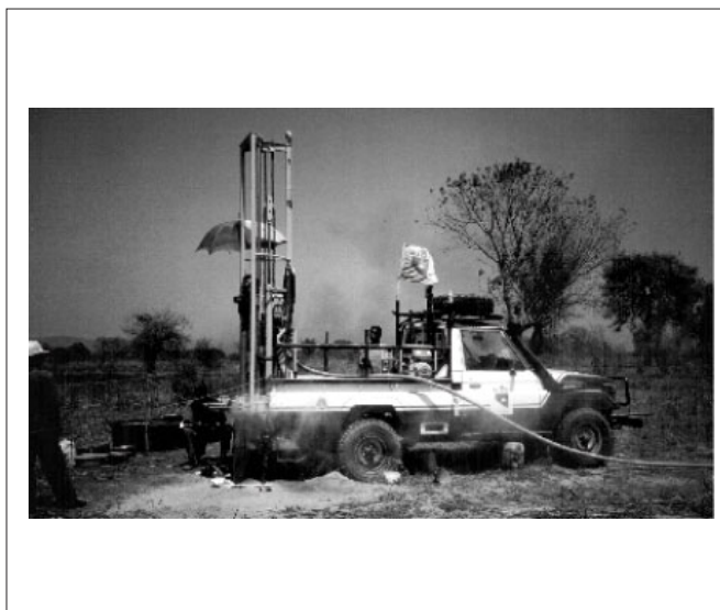
Figure 6: Rig on a vehicle.
