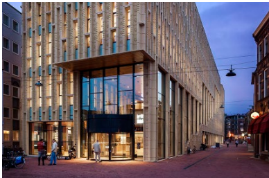
Rozet Arnhem (Neutelings Riedijk Architects, S. Brakkee)
