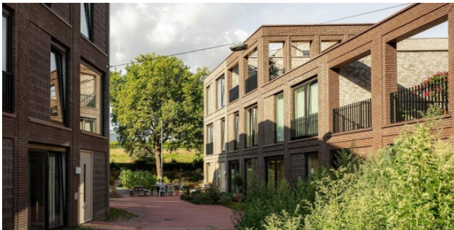
The Hudsons, Rotterdam (Orange Architects, S. v. Damme, S. v. Wettum)
